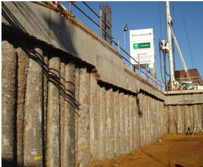
**Figure 7: Example Secant Pile Wall without Fascia**
