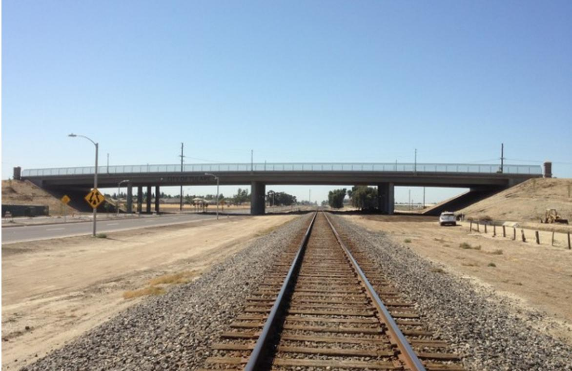
**Figure 4: Overpass Structure; with retaining walls (above), with embankment fill (below)**
