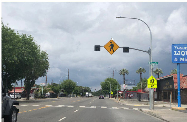
Pedestrian Hybrid Beacon in Modesto CA
