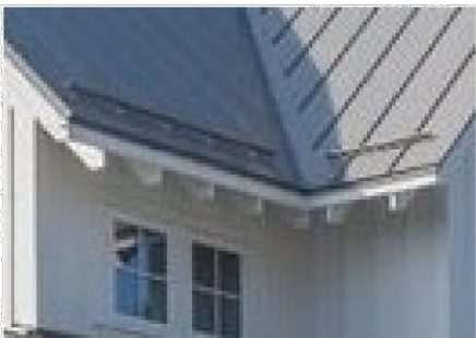
EXPOSED EAVES WITH BEAM TAILS (2 FT OVERHANG & GREATER OVERHANG)
