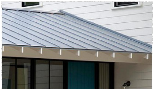
EXPOSED EAVES WITH BEAM TAILS (2 FT OVERHANG & GREATER OVERHANG)
