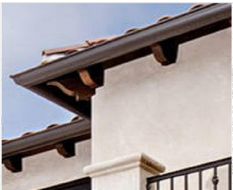
EXPOSED EAVES WITH BEAM TAILS (12 INCHES OR LESS)
