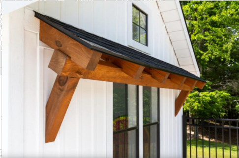
WINDOW AWNING WITH TIMBER BRACKET
