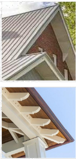
EXPOSED EAVES AND SHAPED RAFTER TAILS (2 FT OVERHANG & GREATER)
